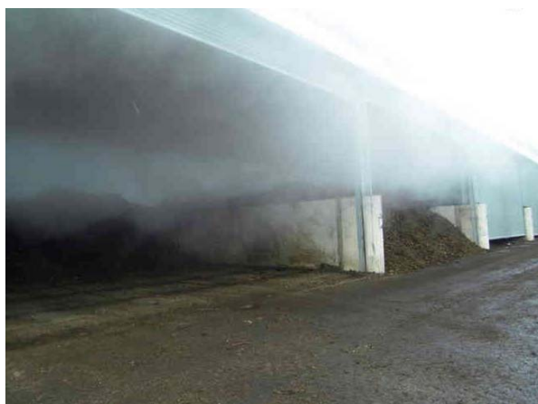
Figure 2: Picture of the fermentation area
